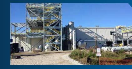
Biochemical processing plant located in Raceland, Louisiana. We provided a wide range of civil and mechanical support services over the span of eight months, including the fabrication, coating and installation of mechanical piping, pipe racks, ducts and flutes, supports and equipment platforms. We also performed pile driving, modifications, hydro testing, commissioning and civil work.
