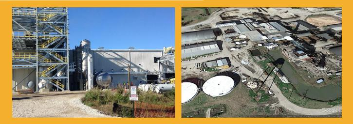
**PROJECT:** Piping and spool fabrication as well as installation of support steel and equipment at a demonstration plant which converts bagasse to xylose.
