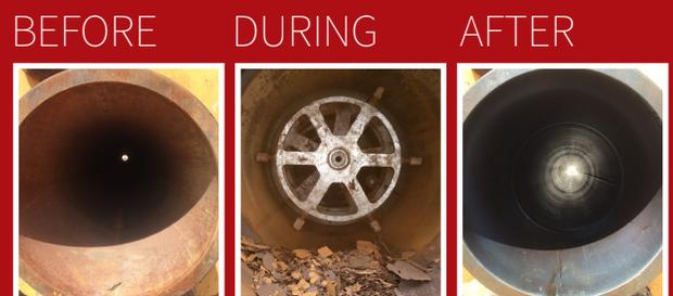
The self-propelled device uses air to move it through the length of the riser and back out, while its brushes oscillate back and forth to clean the debris build up from inside the riser.
